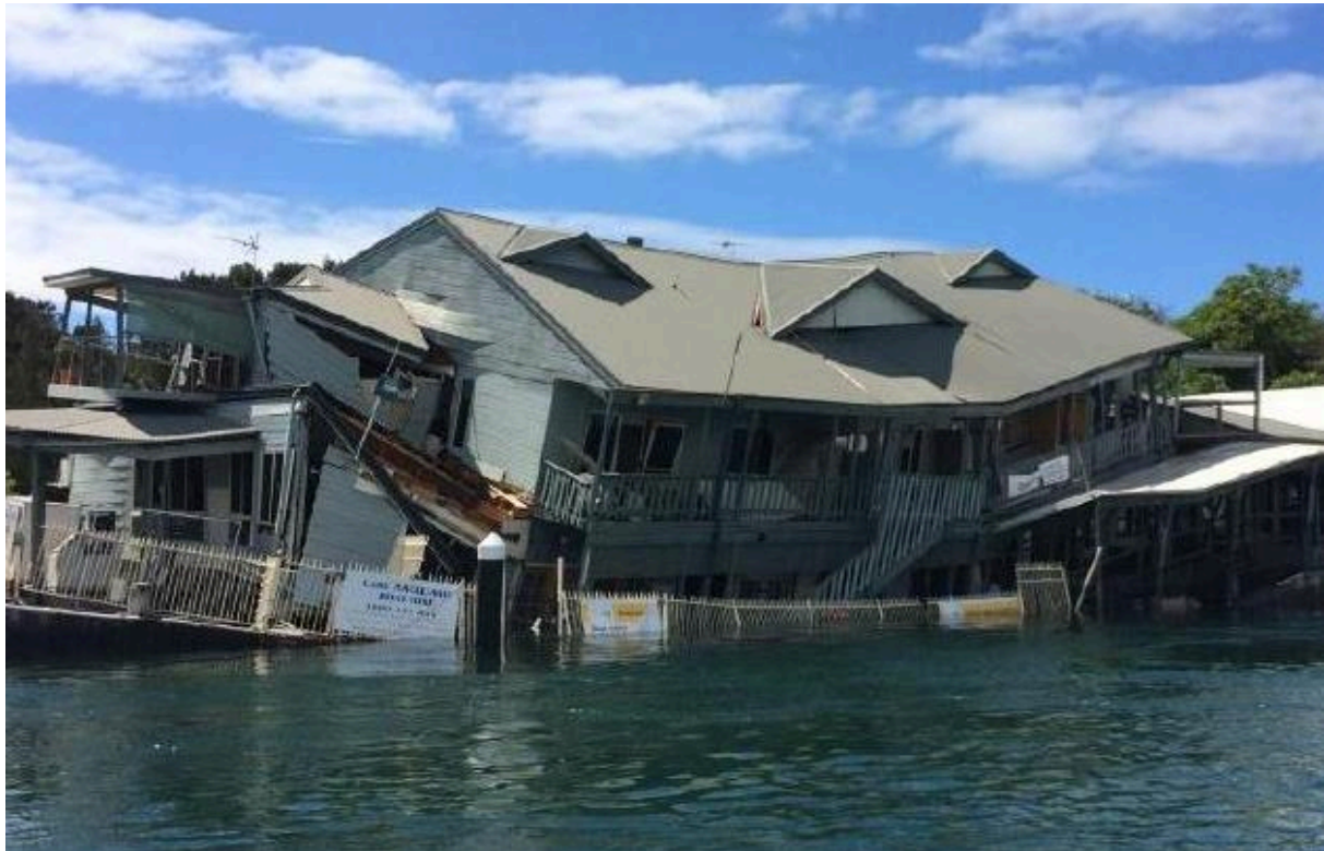
Figure 4 This building at Pelican on the mid north coast of NSW collapsed at 9.45am on 8/2/2016 during calm conditions. It was supported by piles driven into the subaqueous sand at the building's seaward side. Undermining of these piles by an RBF event could explain this sudden collapse.
