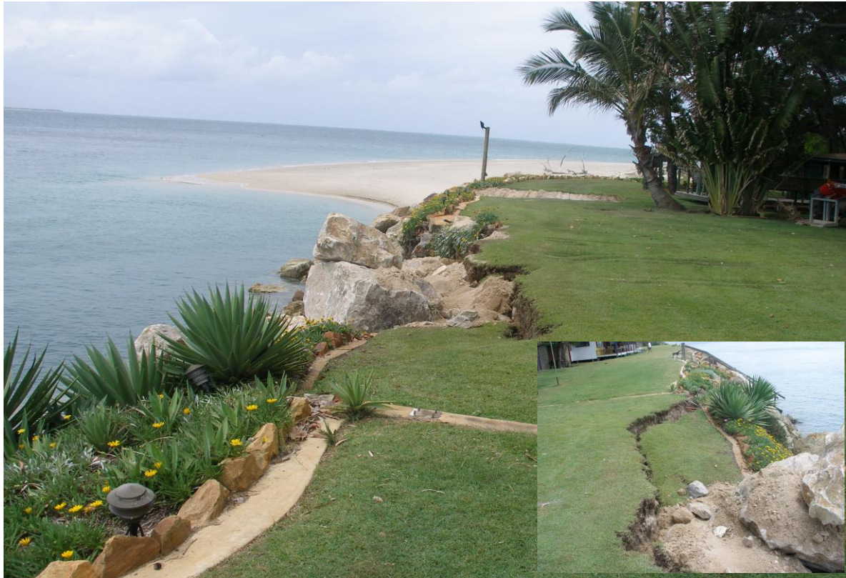
Figure 3. These images show a slump in the riprap 'flow slide barrier' at Amity Point in Queensland after it had been undermined by an RBF event. Repairs by adding new rock have started. The amphitheatre shaped crater in the beach left after the termination of this event can be seen in the background.
