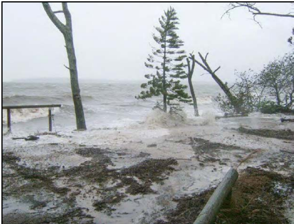
Figure 3-14 Ex TC Oswald storm conditions at Norfolk Beach (Image courtesy of Coochiemudlo Island Coastcare)
