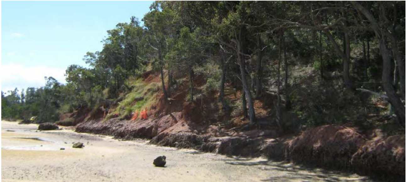
Figure 3-10 Red Cliffs, BMT Site Inspection October 2018
