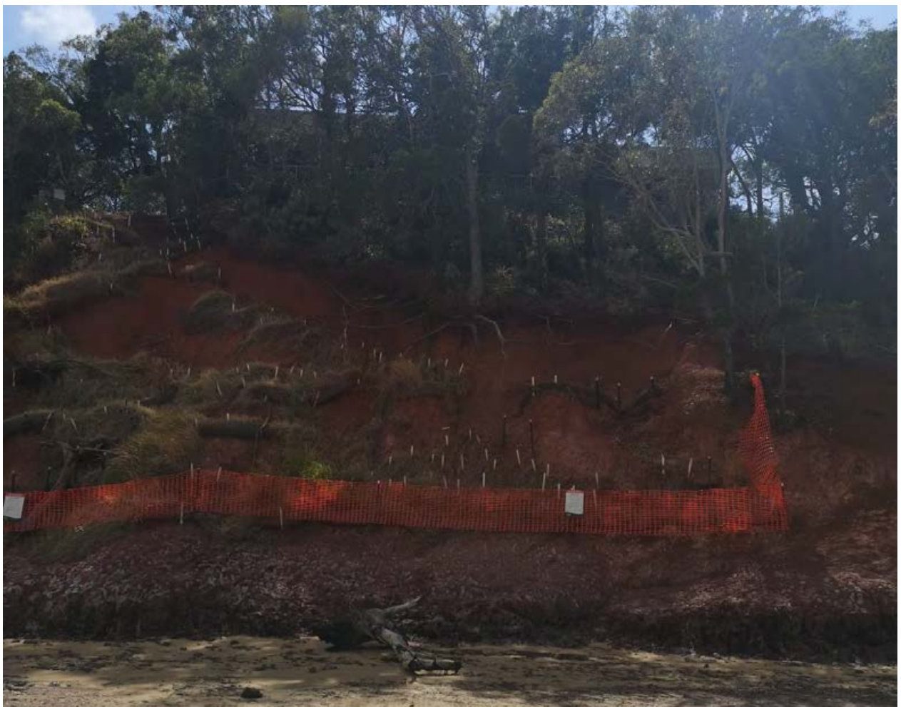
Figure 3-11 Red Cliffs, BMT Site Inspection March 2019
