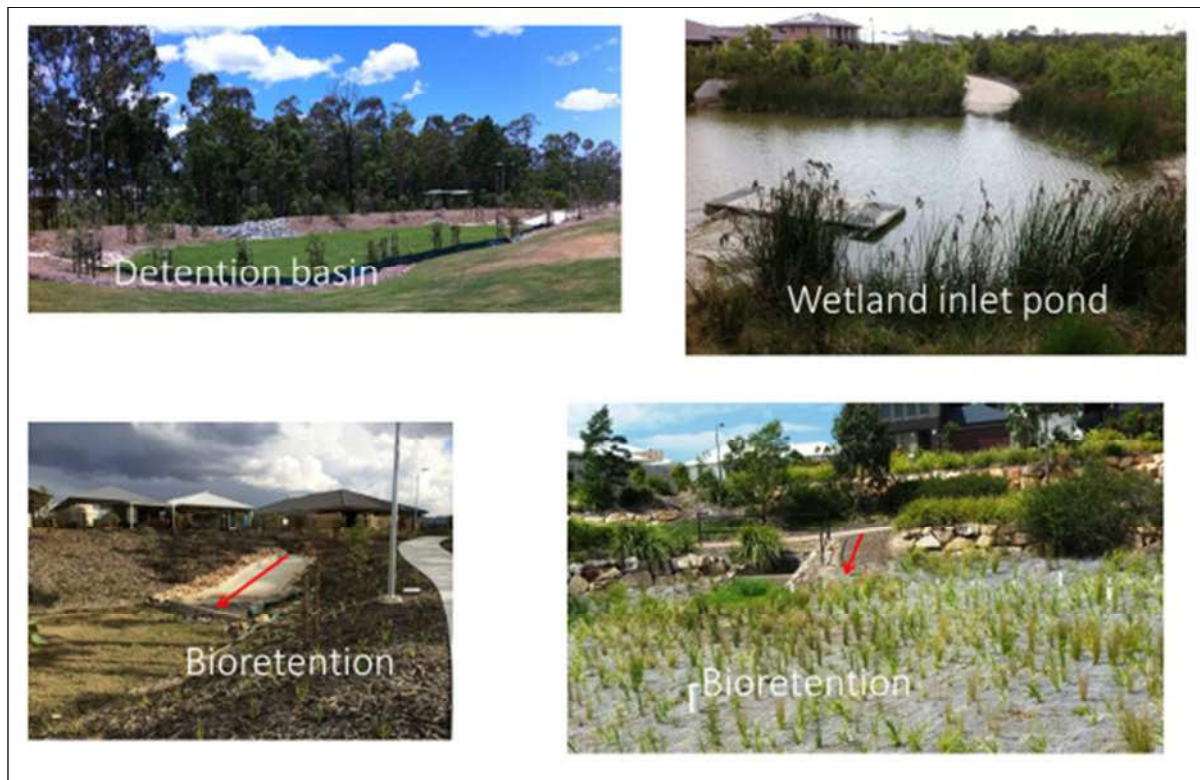
Figure 2.2. Representative photographs showing access options to allow-maintenance works within stormwater ponds/retention basins.
